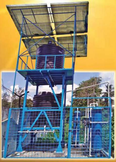
Solar Photovoltaic solution for filtered and purified Drinking Water
